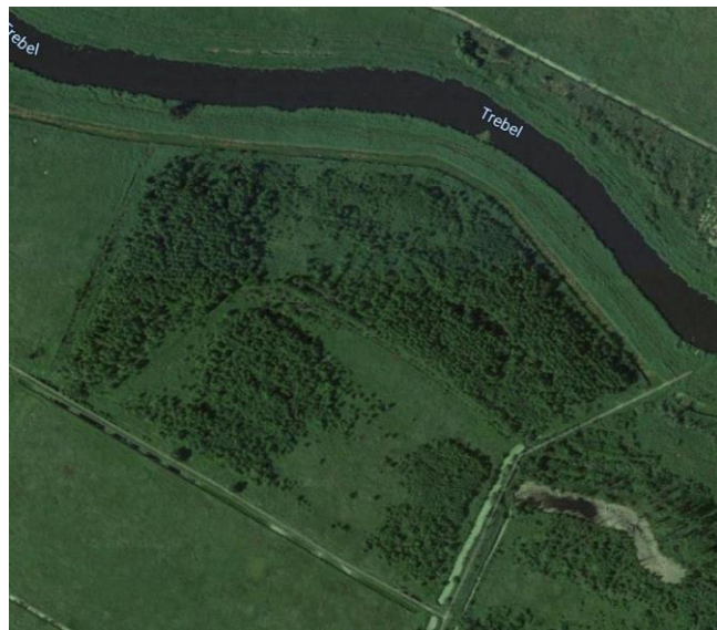
Fig 2: Aerial view of the pilot area 4
