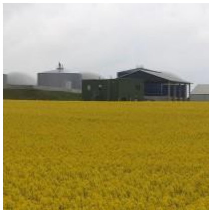
Jordberga Biogas Plant outside Trelleborg (Skåne)
