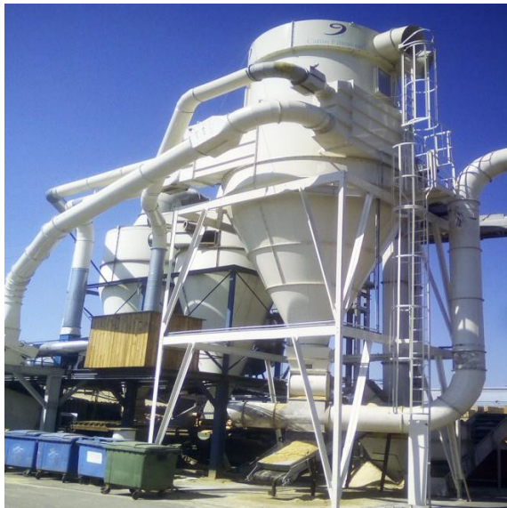
Cyclone dust collector at Wiele Wood Factory
