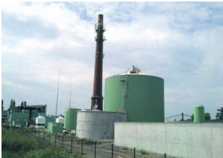
Melno Distillery and Biogas Plant, Poland
