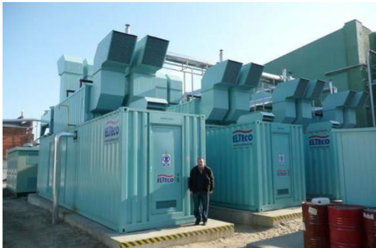
Four cogeneration 400 kWe units at Melno Distillery and Biogas Plant.
