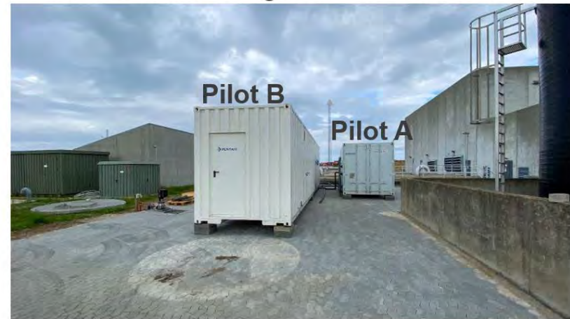
Pilot B: novel ultra tight UF membrane & RO
