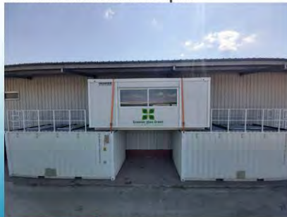
The unit installed in Nafplio
