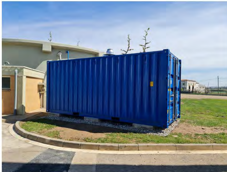
SOFC pilot plant installed in WWTP Lleida
