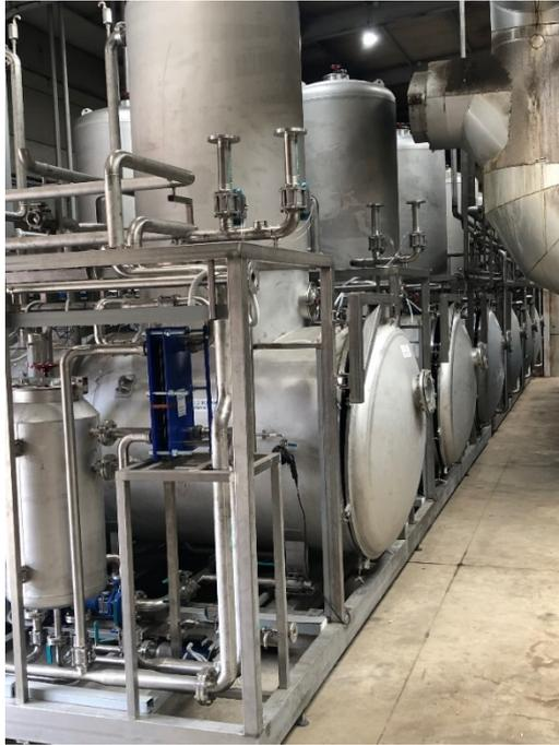
*Photo of the Evaporator-condensator installation at AmPower (Pittem, Belgium).*
