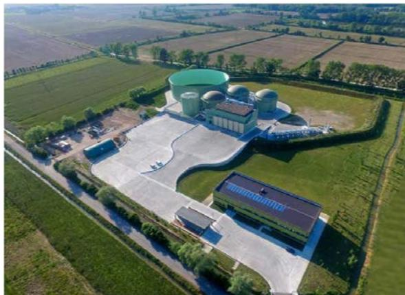
**Acqua & Sole S.r.l.**, a thermophilic anaerobic digestion plant in Vellezzo Bellini (30 km south of Milan), Pavia, Lombardy, Italy, in operation since 2016 with a total annual substrate processing capacity of 120,000 tonnes. Processing municipal sewage sludge and source separated domestic food waste.
