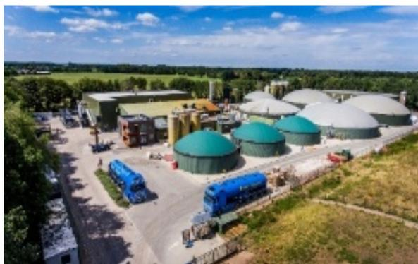
**Groot Zevert Vergisting B.V.**, a mesophilic anaerobic digester plant in Beltrum (35 km southwest of Enschede), Achterhoek Region, Province Gelderland, The Netherlands, in operation since 2004 with a total annual substrate treatment capacity of 135,000 tonnes. Processing pig manure and residues from agro-food industry.
