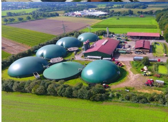
**BENAS GmbH**, a thermophilic anaerobic digestion plant in Ottersberg (40 km east of Bremen), Lower Saxony, Germany, in operation since 2006 with a total annual substrate processing capacity of 174,000 tonnes. Processing corn silage, plant residues and poultry litter.
