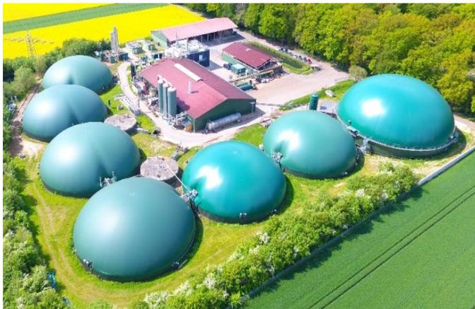
**BENAS GmbH**, a thermophilic anaerobic digestion plant in Ottersberg (40 km east of Bremen), Lower Saxony, Germany, in operation since 2006 with a total annual substrate processing capacity of 174,000 tonnes. Processing corn silage, plant residues and poultry litter.
