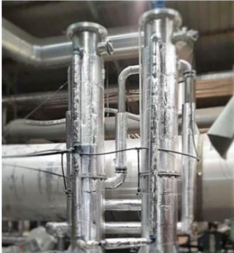
Figure 2: Pilot Plant FiberPlus
