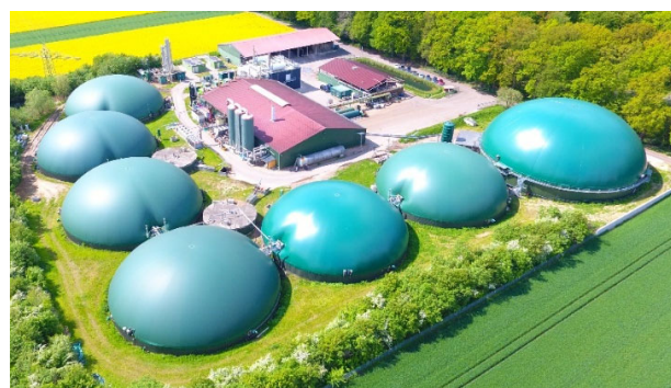
Figure 1. Aerial photo of the demonstration plant BENAS.
