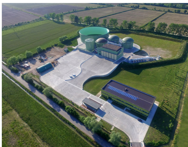
Figure 1. Aerial photo of the demonstration plant Acqua & Sole.
