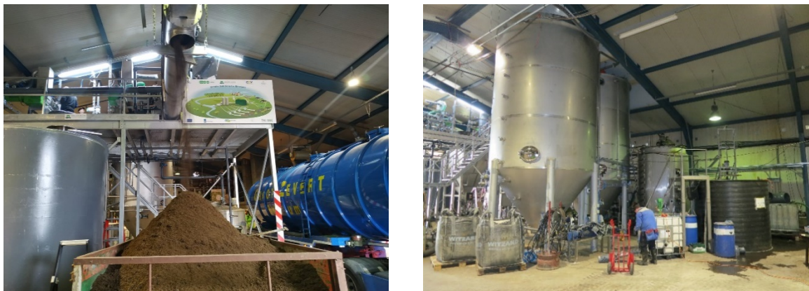
Figure 2-2 Photos of process units of the RePeat system at the demonstration plant GZV (left; screw presses and collection of low-P organic soil improver. Right; stainless steel precipitation tank and settling tank for precipitation and dewatering of precipitated P salts).
