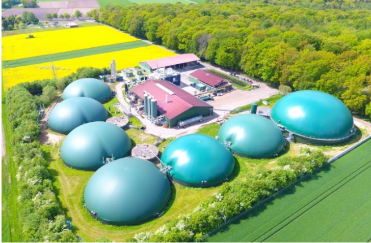
Figure 5-2 Aerial photo of the demonstration plant BENAS (2019).
