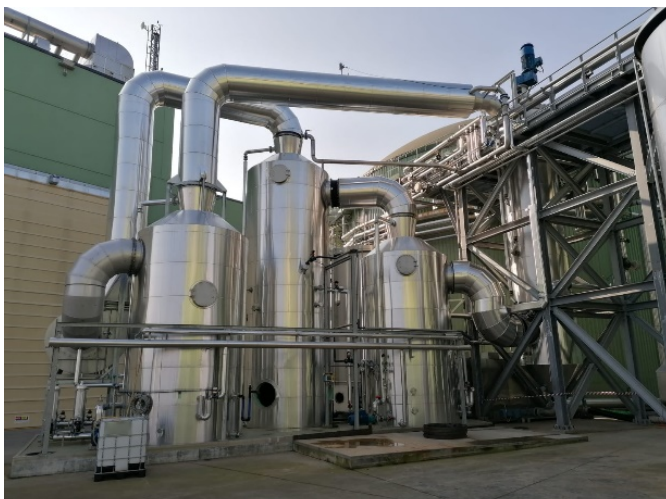
Figure 4-2 N absorber installed at the demonstration plant Acqua & Sole (2020).
