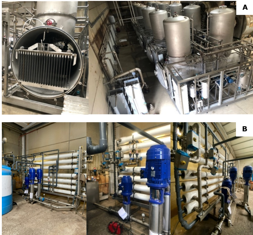
Figure 3-2 Photos of the vacuum evaporator (a) and reverse osmosis unit (b) of the demonstration plant Am-Power.
