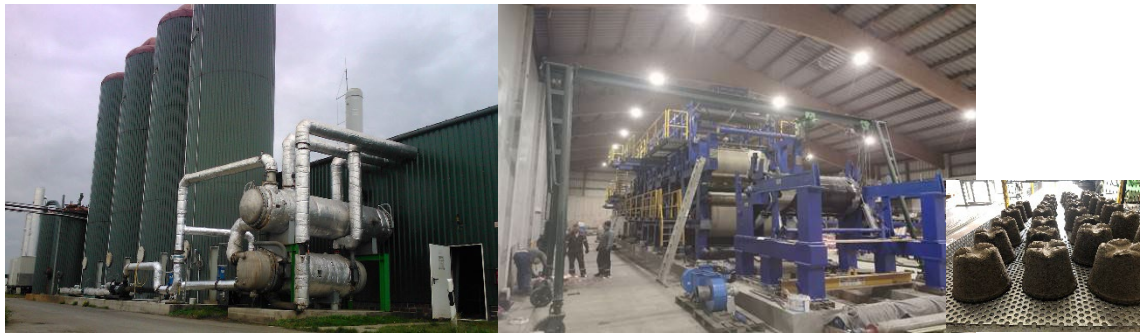
Figure 4.8 The NRR installation at BENAS; N stripping towers, paper producing machine and pots produced from recovered fibres.
