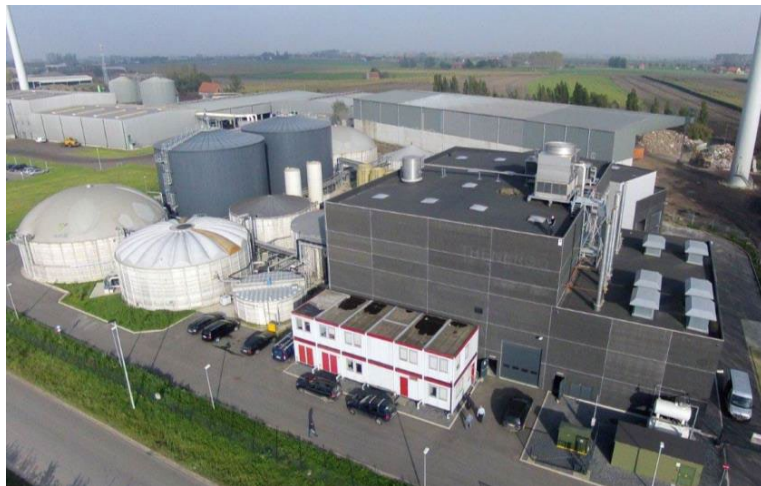
Figure 4.12 Aerial photo of the demonstration plant Waterleau NewEnergy (2019).
