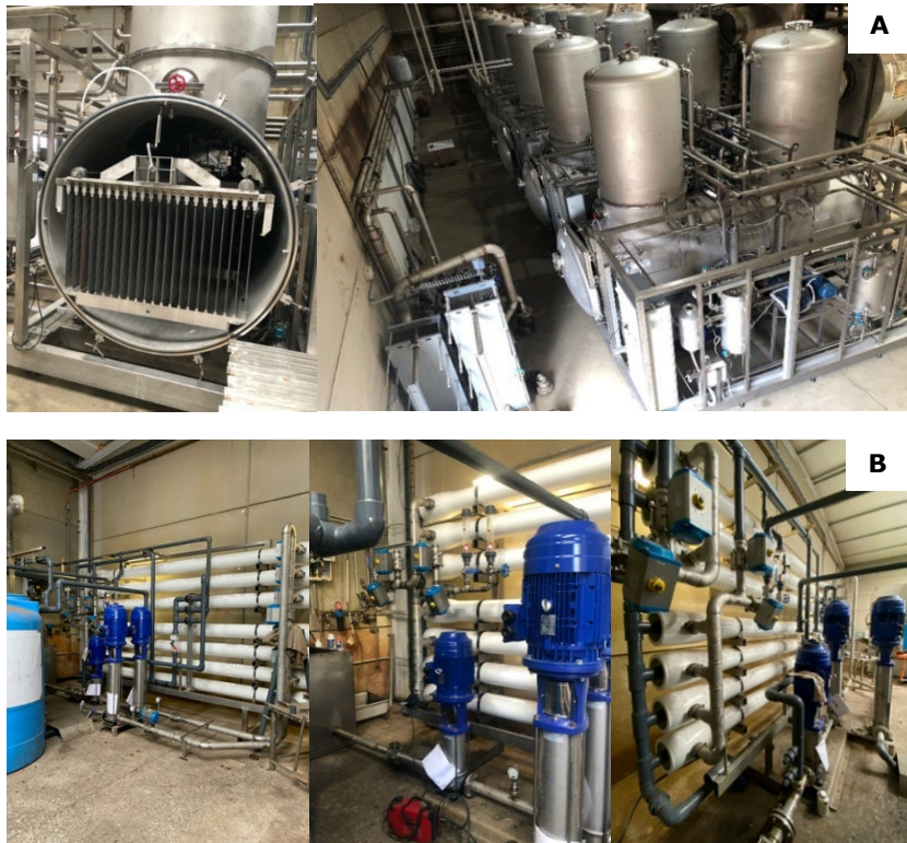
Figure 4.5 Photo of the new evaporators at Am-Power (upper) and RO installation for treatment of the condensate of the evaporator (below)
