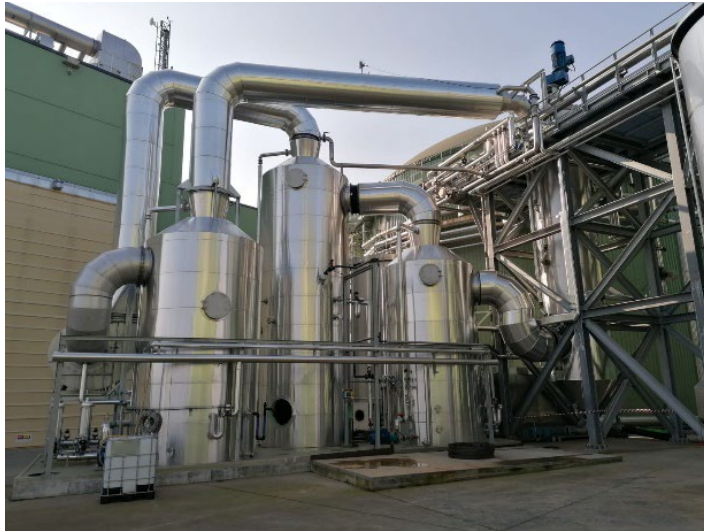
Figure 4.10 The new N stripper at Acqua&Sole (Italy)
