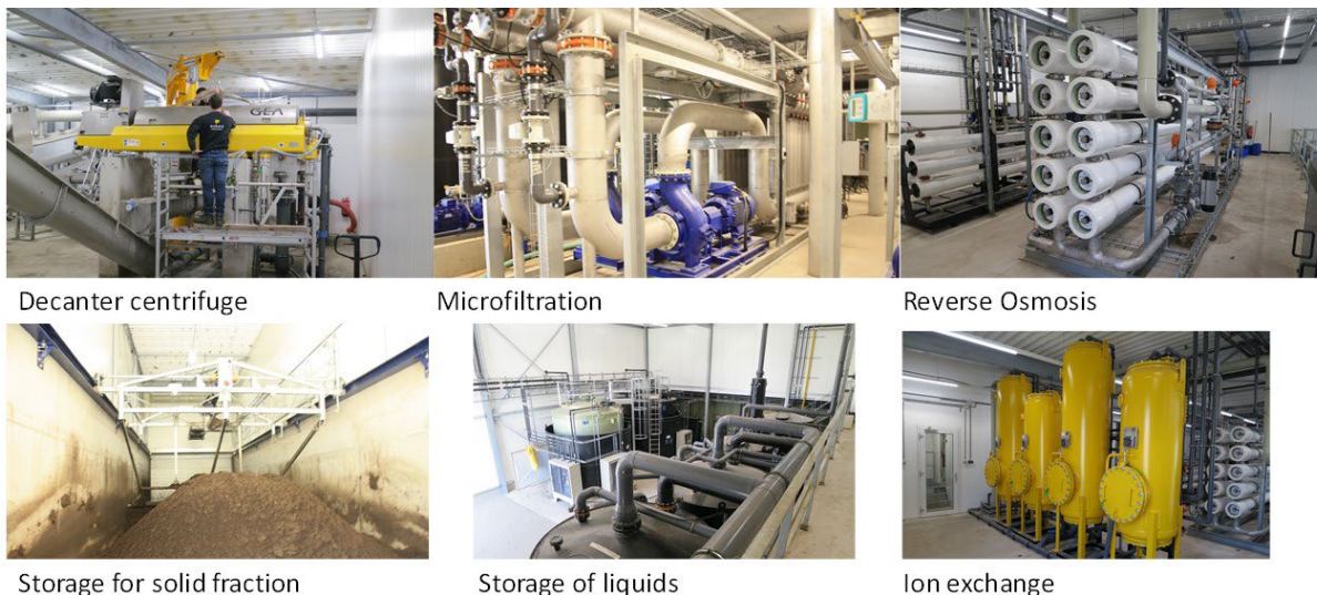
Figure 4.3 The new GENIUS installation at GZV
