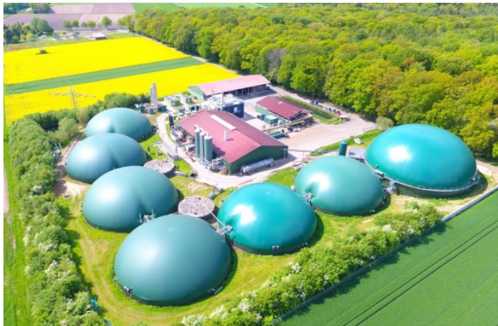
Figure 4.7 Aerial photo of the AD plant of BENAS (Germany) including the N stripping towers.
