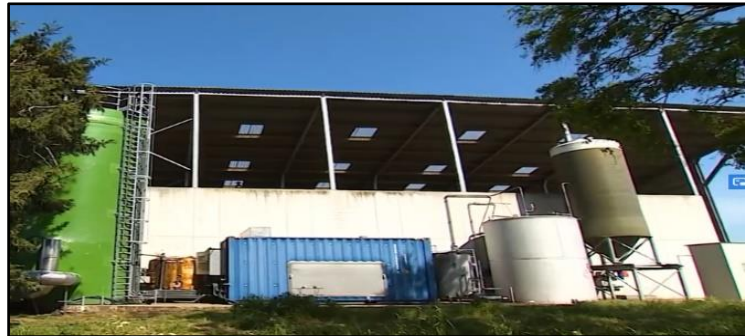
Figure 1 Ammonia stripping/scrubbing installation plant at Detricon site (Gistel, Belgium).
