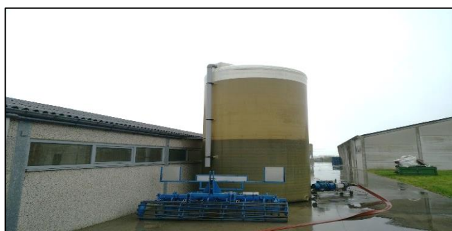
Figure 1 Ammonia scrubbing unit at pig farm in Merkem (Belgium).
