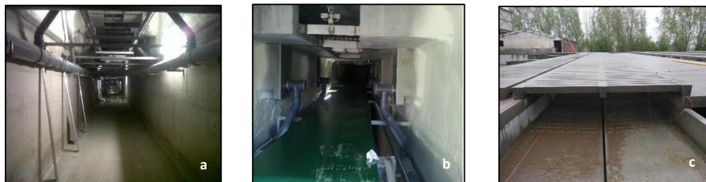
Figure 1 The VeDoWS system for manure separation from Vermeulen Construct: a) pipeline which collects urine from all the stable units; b) conveyor belt to transfer the solid manure from the slatted floor to the manure storage area; c) gutter for urine collection.
