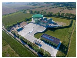
**Acqua e Sole S.r.l.**, a thermophilic anaerobic digestion plant in Vellezzo Bellini (30 km south of Milan), Pavia, Lombardy, Italy, in operation since 2016 with a total annual substrate processing capacity of 85,000 t. Processing municipal sewage sludge and source separated domestic food waste.
