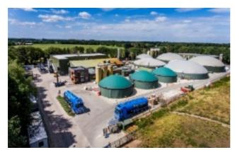
**Groot Zevert Vergisting B.V.**, a mesophilic anaerobic digester plant in Beltrum (35 km southwest of Enschede), Achterhoek Region, Province Gelderland, The Netherlands, in operation since 2004 with a total annual substrate treatment capacity of 135,000 t. Processing manure and biowaste.
