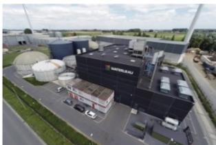
**Waterleau BV,** a mesophilic anaerobic digestion plant in Ypres (80 km west of Ghent), West-Flanders, Belgium, in operation since 2012 with a total annual substrate treatment capacity of 120,000 t. Processing manure and biowaste.
