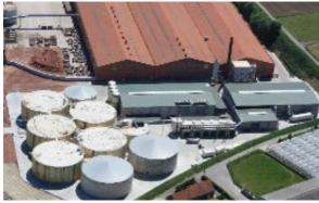
**AM-Power BVBA**, a thermophilic anaerobic digestion plant in Pittem (40 km west of Ghent), West-Flanders, Belgium, in operation since 2011 with a total annual substrate processing capacity of 180,000 t. Processing biowaste and manure.
