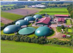
**BENAS GmbH**, a thermophilic anaerobic digestion plant in Ottersberg (40 km east of Bremen), Lower Saxony, Germany, in operation since 2006 with a total annual substrate processing capacity of 174,000 t. Processing corn silage, plant residues and poultry litter.
