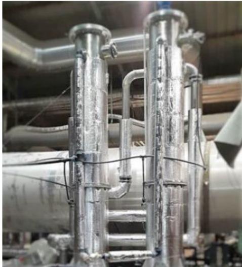
Figure 2.2: Pilot Plant FiberPlus
