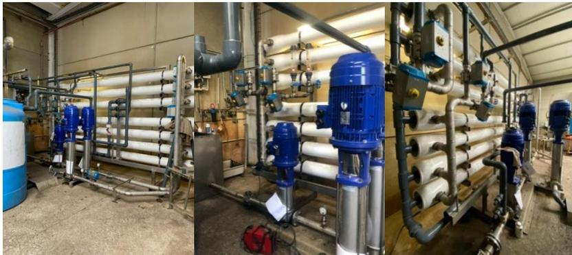
*Figure 2.3 The new reverse osmosis unit installed at the demonstration plant AM-Power (2020).*
