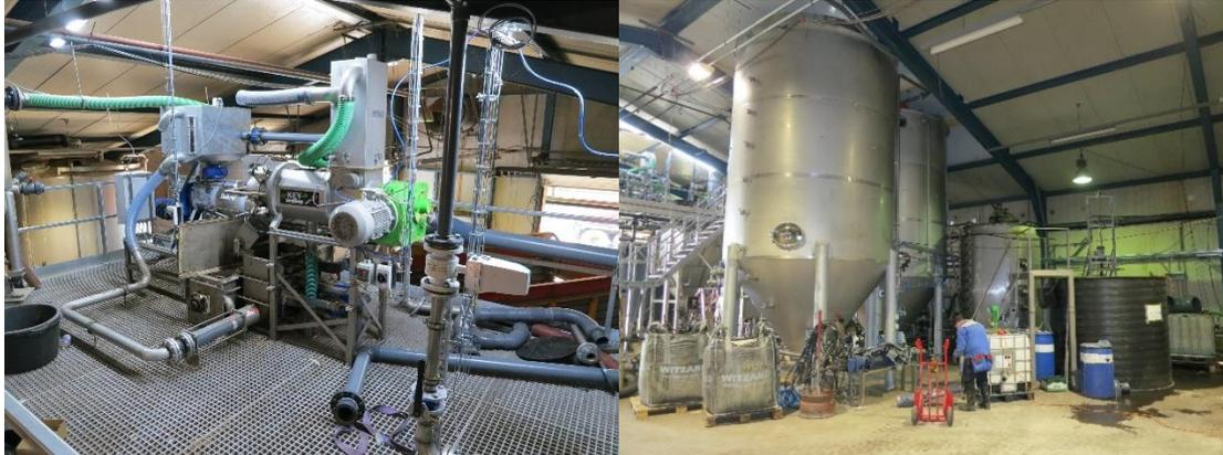
Figure 1.1 Photos of the new RePeat installation at Groot Zevert Vergisting (left; screw presses, right; stainless steel settling tank, stainless steel precipitation tank and a black buffer tank).
