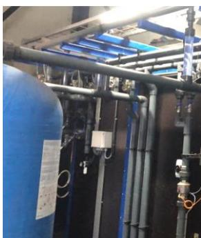
*Figure 2.4 The new ion exchanger installed at the demonstration plant AM-Power (2020).*
