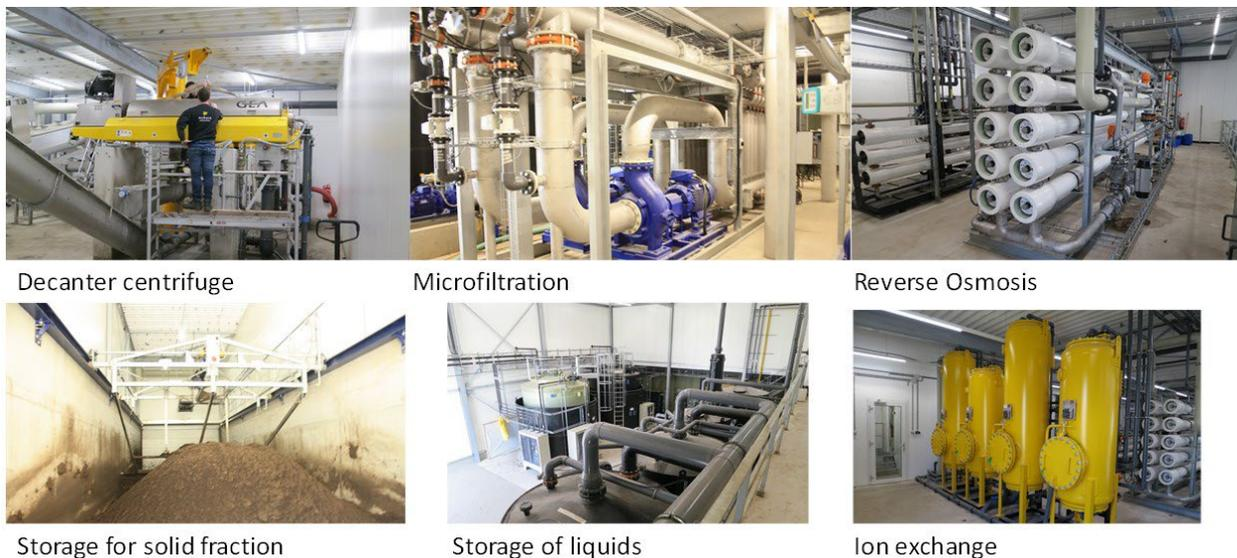
Figure 1.1 Photo's of the new GENIUS installation for the production of solid fraction, NK concentrate and clean water from digestate
