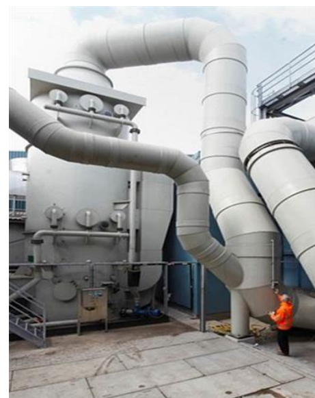
Figure 2: Acid air washer for Ammonium sulphate production.
