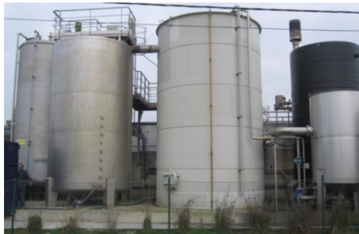
Figure 15: Struvite recovery reactors (right: stripping reactor, left: crystallization reactor).
