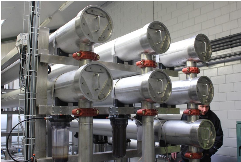
Figure 15: Picture of a reverse osmosis installation.
