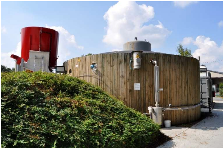
Figure 1: Small-scale Anaerobic Digester
