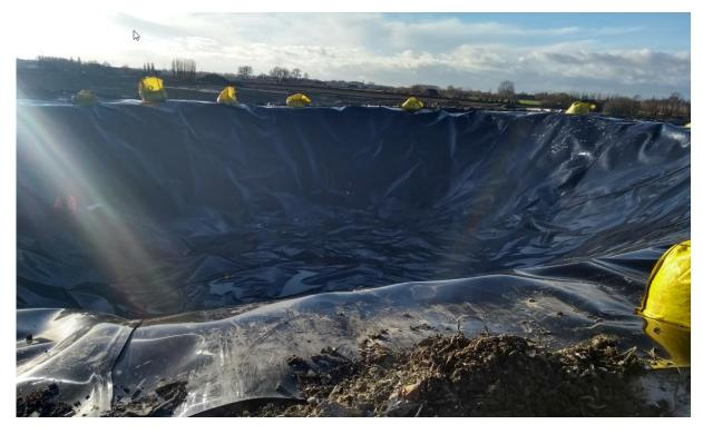
HDPE film is used as a liner and top cover to create a closed reactor.
