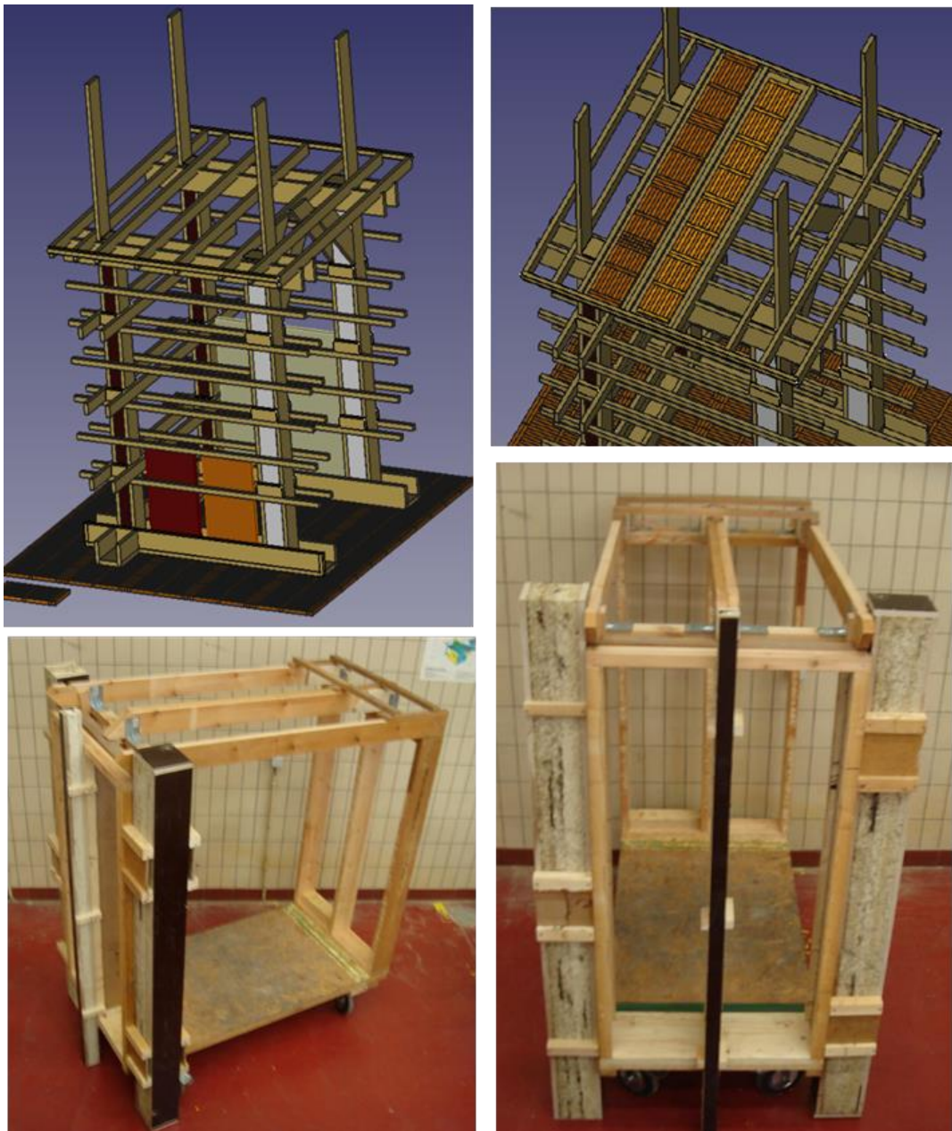
Figure 177: HOGENT demo-unit integrating and showcasing the different biocomposite prototypes of building and landscaping products. CAD design drawings showing the positioning of the mineral beams blocks and biobased plate and sheathing materials, and the demo-unit in construction (indoor).
