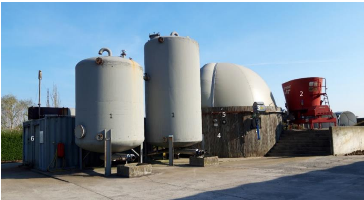
Figure 3: Overview of the biogas pilot plant at Inagro: (1) Silage tanks to store and feed liquid fraction of pig slurry; (2) Screw press to feed the VeDoWS manure and the roadside grass; (3) Mixer; (4) Reactor; (5) Air injection for desulfurization; (6) CHP; (7) trench silo for VeDoWS.
