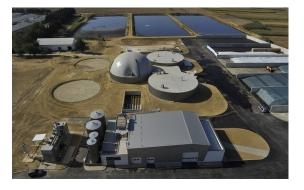
At first, the Biogas Plant Gradec was built as a 1  $MW_{el}$  plant with a CHP but was advanced with two separate hydrolysis tanks and a 2<sup>nd</sup> CHP in 2015. Production with 2 MW capacity started in the 4<sup>th</sup> quarter of 2015.
