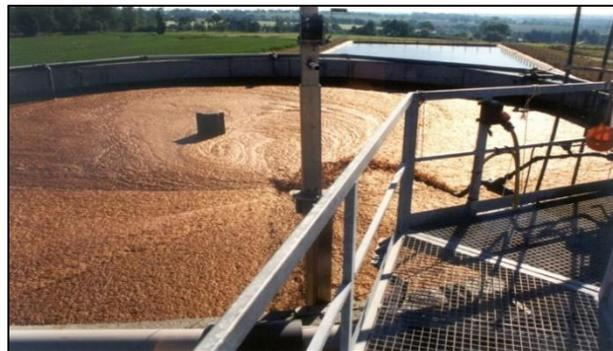
**Figure 10.** Biological nitrification/denitrification tank (VCM, n.d.)
