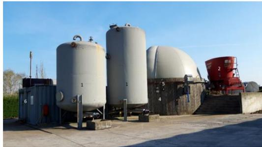
The installation used was a classic CSTR reactor (200 m<sup>3</sup> with a filled volume of approximately 150 m<sup>3</sup>), with an electrical power of 31 kW, which is controlled by Inagro in the mesophilic temperature range ( $\pm 38$  ° C). The biogas is burned in a combined heat and power unit (CHP) after water vapor and sulfur are removed via a condensation step and biological desulfurization.
